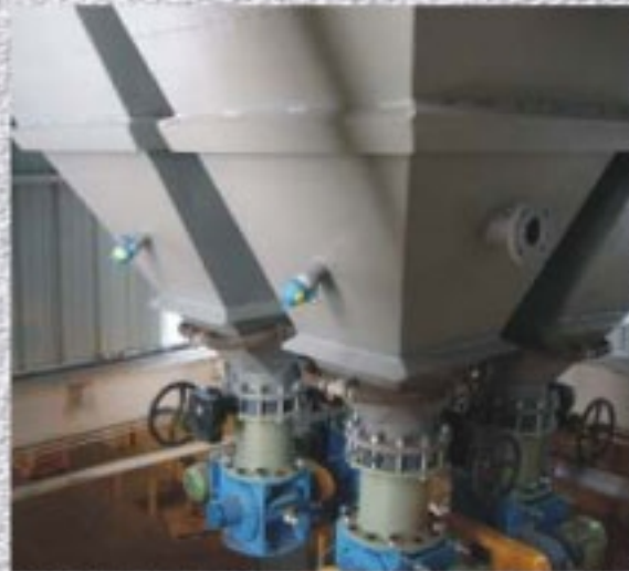
Batch Hopper with Rotary discharge Valve
